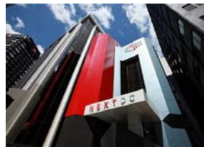
Data Centres Next DC, NSW
